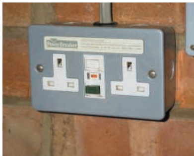
A metal-clad RCD suitable for workshop use.
