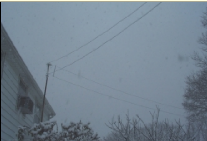
The shack end of the installation. The coax runs perpendicular to the antenna down the wooden pole and into the window to the right of the air conditioner.
