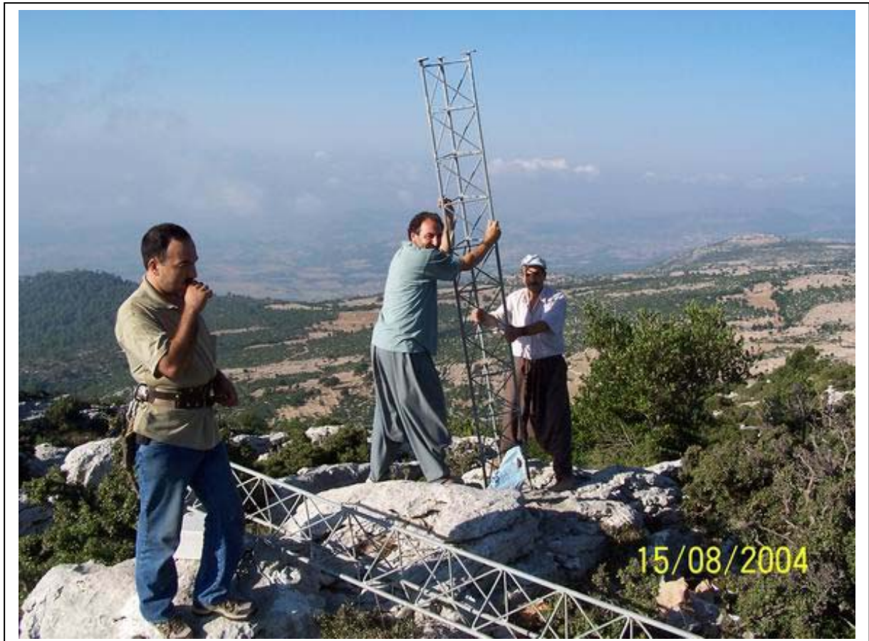
On top of the hill finally. The tripod mast (ready to be erected) was carried and the concrete base was poured between the rocks by KASIM and MEHMET three weeks ago. Looking South-West at the direction of Mersin and Cyprus. The elevation of the RX site is 997 meters and the length of the mast is 6 meters.
