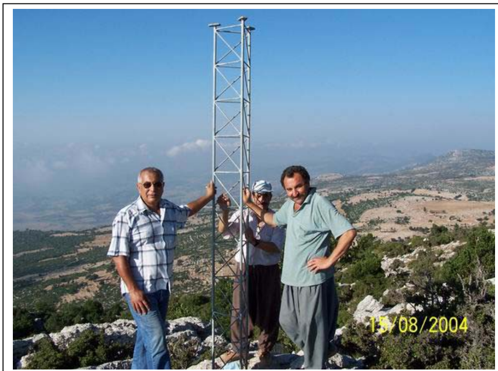
On top of the hill finally. The tripod mast (ready to be erected) was carried and the concrete base was poured between the rocks by KASIM and MEHMET three weeks ago. Looking South-West at the direction of Mersin and Cyprus. The elevation of the RX site is 997 meters and the length of the mast is 6 meters.
